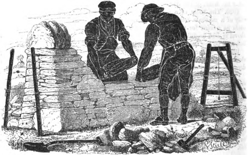
THE BUILDING A DRY-STONE DYKE.
