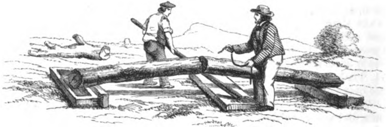
PREPARATION OF THE TIMBER FOR BOCCHERIE'S METHOD OF PRESERVING IT.
