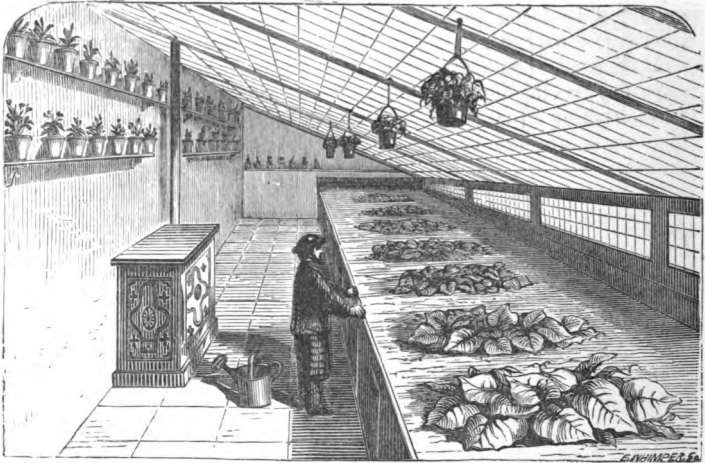
INTERIOR OF LEAN-TO HEATED BY MUSGRAVE'S SLOW COMBUSTION STOVE.
